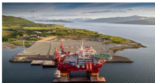
Grøtsund quay 1 with ro-ro ramp
